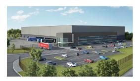
A 2022 DTZ ESG case study is the 148,240 Sq. Ft / Industrial / Distribution facility at Trafford Park, Manchester. This asset improvement scheme set to achieve BREEAM Excellent and an EPC A+ rating through the incorporation of 1,700 sq m of PV panels (generating 295,700 kWh per annum), 14 EV individual charging points, a rainwater harvesting tank and half hourly water metering and sub-metering.
