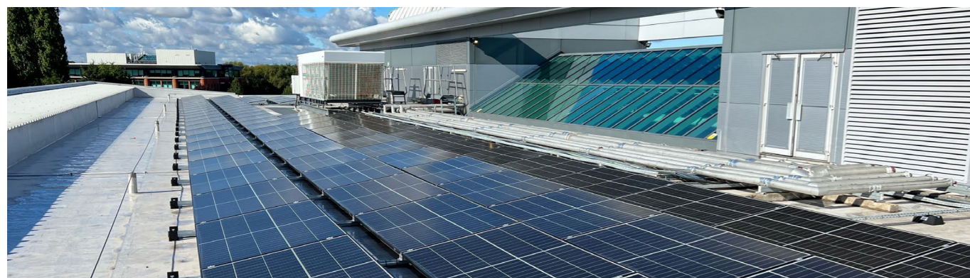
Installation of solar panels at T3, Solihull UK
