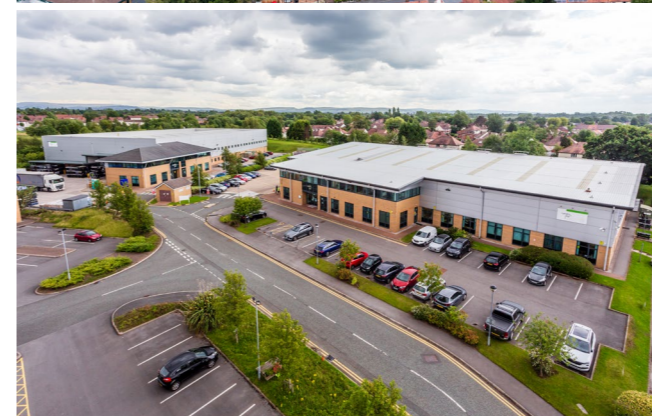
Stockport - Prior to PV installation
