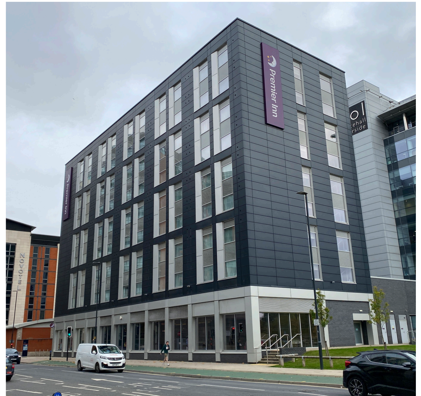
Premier Inn, Leeds UK
